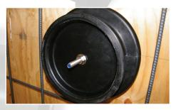
Slide second locator cap through (threaded rod\*), use fender washer and fasten nut until locator caps and sleeve are locked in place. Check to make sure sleeve is square to form.
