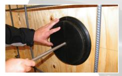
Extend (threaded rod\*) through form and first locator cap and (threaded nut\*) on the back side of form.
