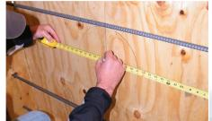
Using a tape measure, pull measurements from the horizontal and vertical positions to locate the center of the Infinity<sup>®</sup> wall sleeve.
